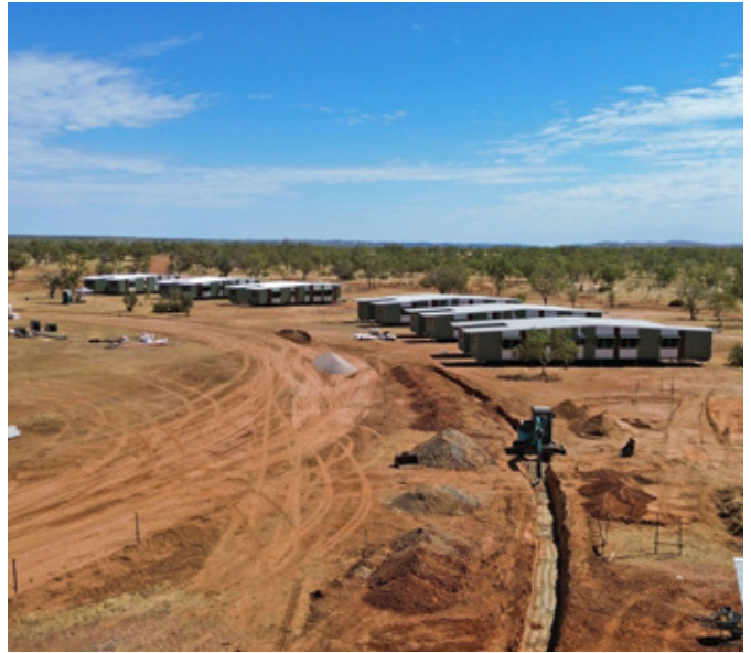
Manjali Studio School site during construction August 2024. Image owned by HMA.
